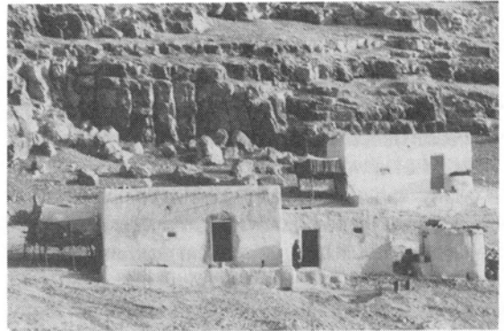
Plate 6 Stone and mud plaster houses and sleeping platforms of wood in the village of Joussef Pasha, with cliff of well-bedded upper unit calcarenite behind.
