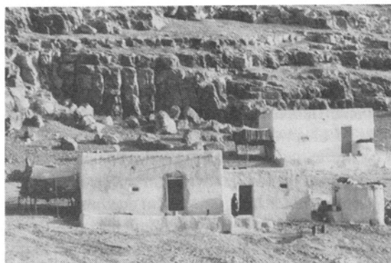
Plate 6 Stone and mud plaster houses and sleeping platforms of wood in the village of Joussef Pasha, with cliff of well-bedded upper unit calcarenite behind.
