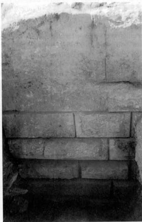
Illustration 4: Foundation blocks, north-east corner, Room 9
