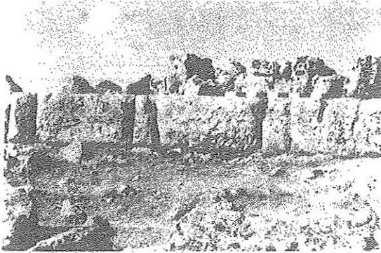
Pl. 3: Header and Stretcher construction of City Wall
